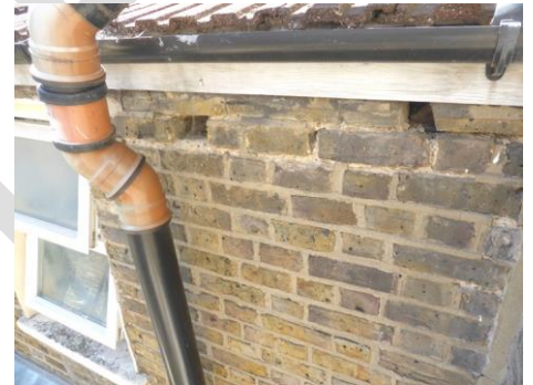
Gaps in rear addition wall
