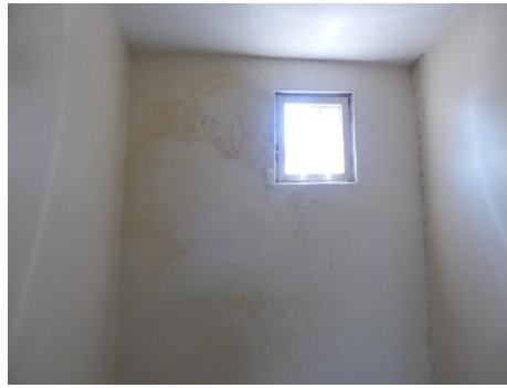
Penetrating damp hall rear wall
