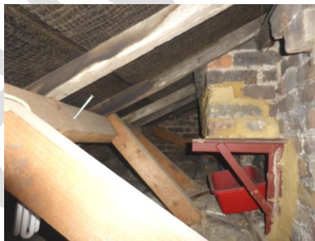
Rear addition roof space and gallows brackets
