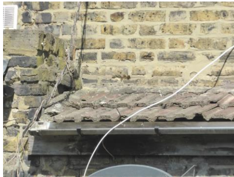
Kitchen roof and defective parapet
