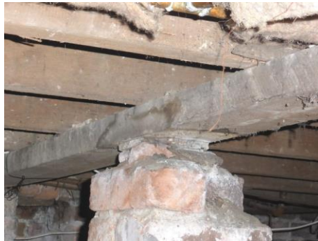
Damp cellar joist above brick pier
